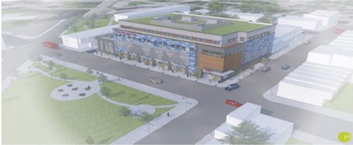
View looking north east
