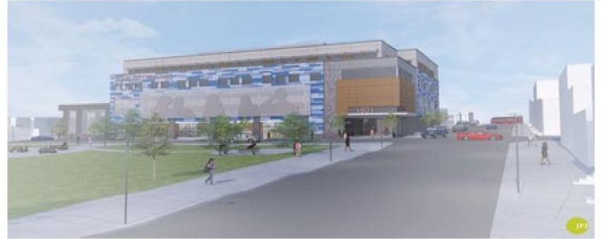
View looking east down Oliver
