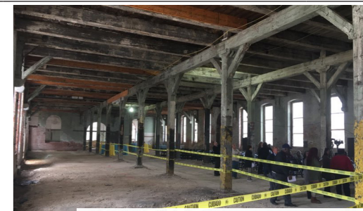
HOEN BUILDING STABILIZATION
