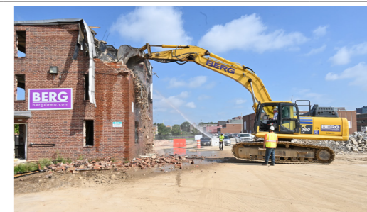
PERKINS HOMES DEMOLITION
