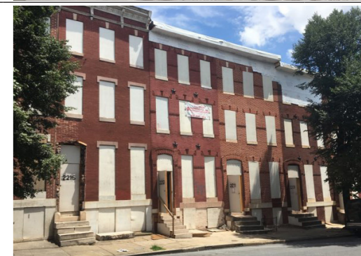
DRUID HILL AVE STABILIZATION
